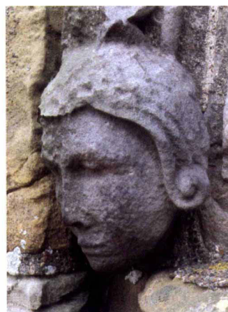
Figure 7 Badly eroded gargoyle at Whitby Abbey
