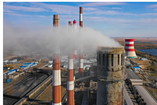
CO 2 is emitted by industrial processes
