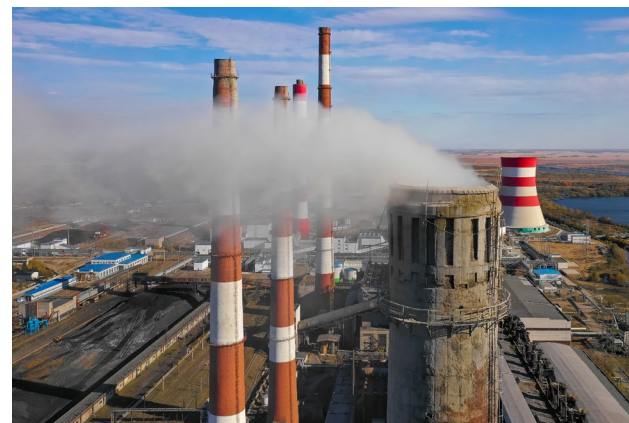
CO 2 is emitted by industrial processes
