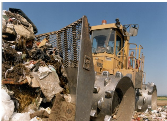
Bulldozer at work on a landfill site (Photograph courtesy of Biffa)
